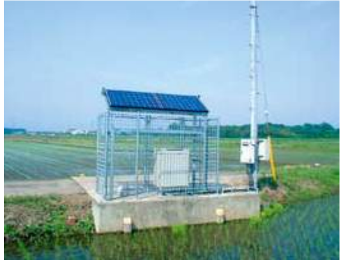
Cathodic protection using solar power
