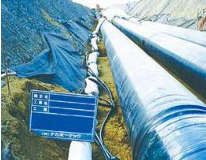
Pipeline corrosion protection with magnesium alloy anodes
