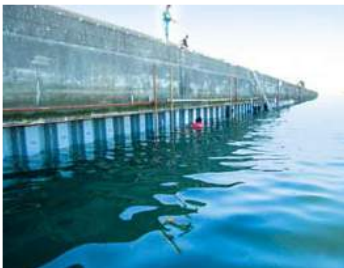
The application of “PTC” system to steel sheet piles
