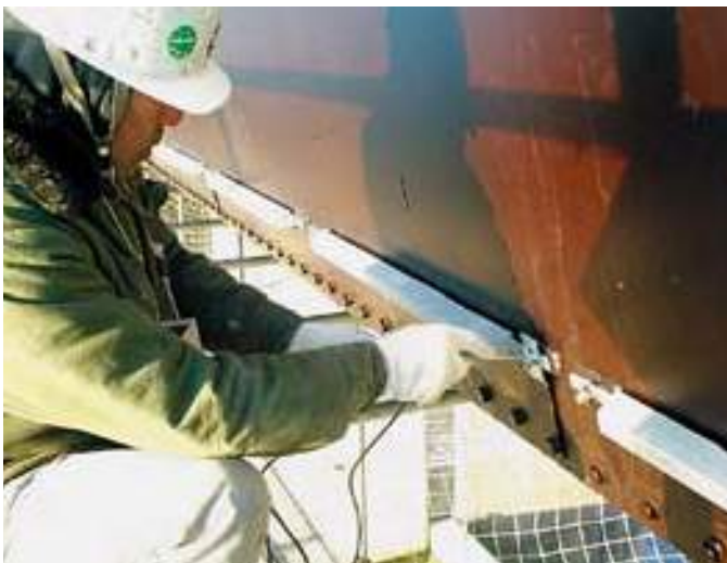
Magnesium alloy anodes installed on a weir facility
